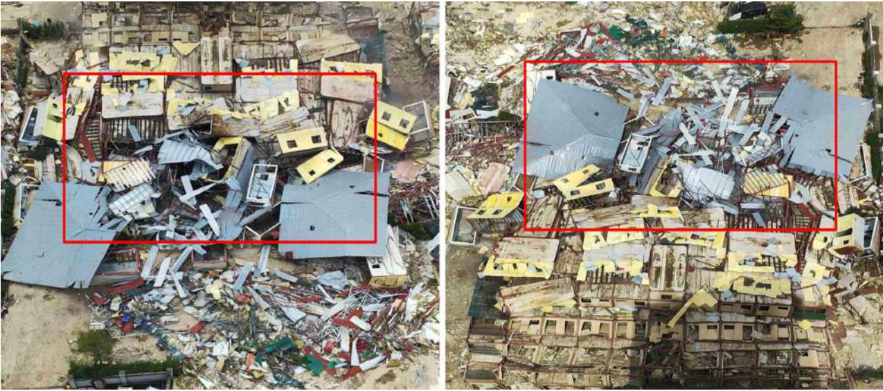
The illegal 17-storey building in the Shwe Kokko area of Myawaddy District, Kayin State, where online scam and illegal gambling operations were conducted.
