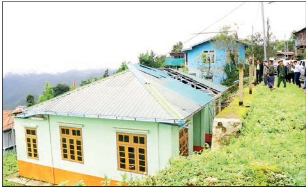
The deputy minister and officials inspect the repair work at staff housing in Tiddim, Chin State.
