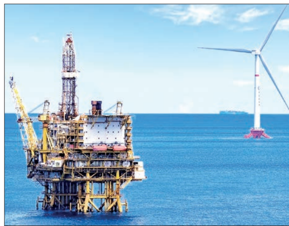
Haiyou Anlan, a floating tension-leg platform wind turbine developed by CNOOC, situated next to an oil platform. PHOTO: CGTN
