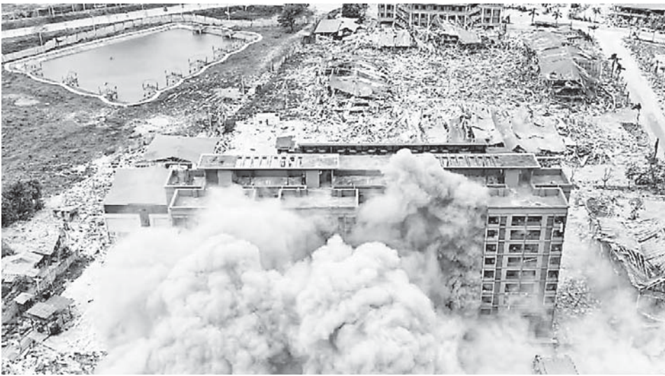
Online scam and gambling buildings being blown up in KK Park.
