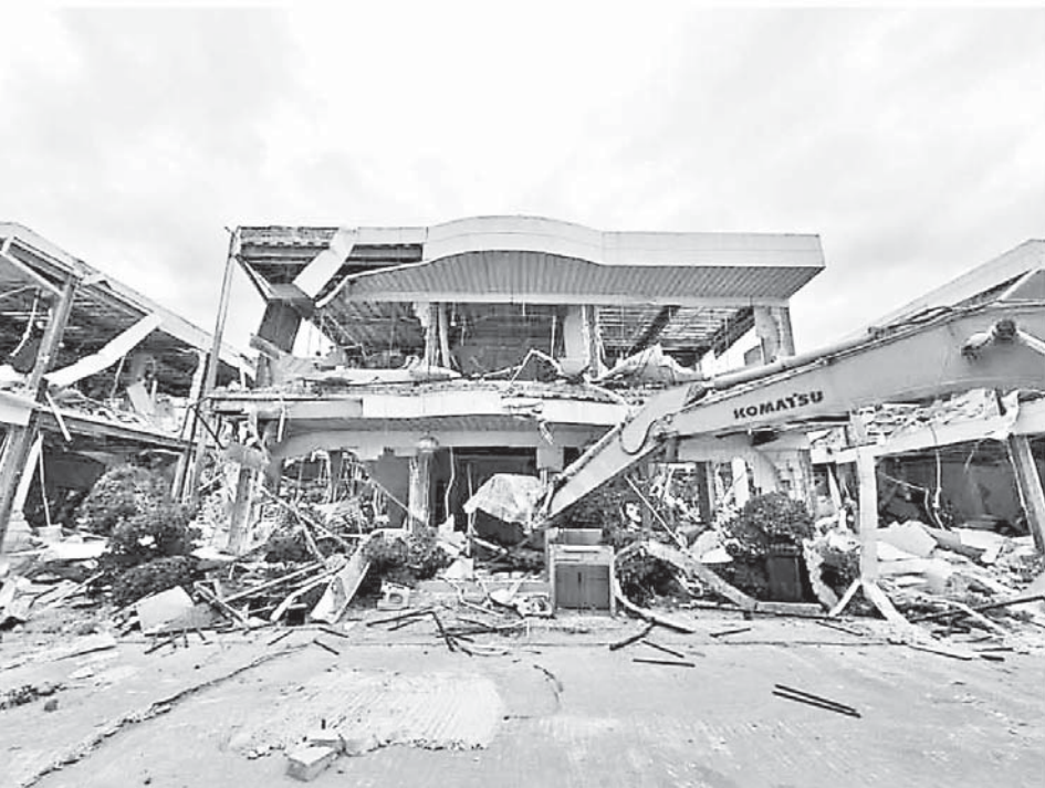
Demolition of an online scam and gambling building with the use of heavy machinery in KK Park.
