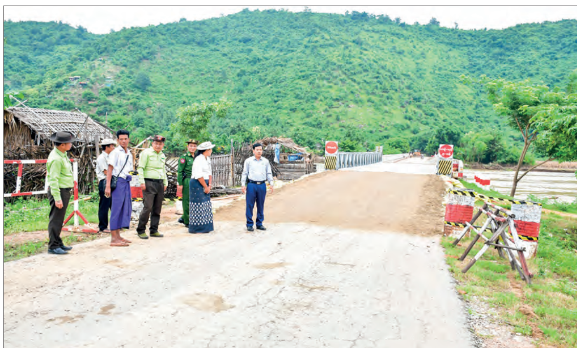
Nay Pyi Taw Council Chairman U Than Tun Oo looks into the construction of a 80-foot two-layer temporary bailey bridge yesterday at the site of Zeephyupin Village bridge across the Paunglaung River damaged by water erosion.
