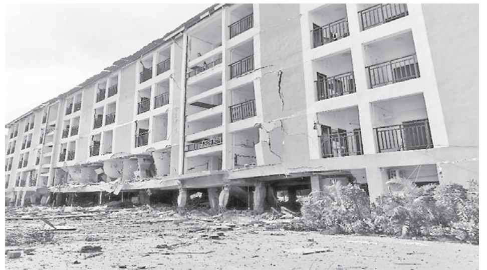
Photo shows a five-storey residential building that was blown up with explosives.
