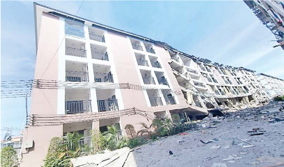
Photo shows a five-storey residential building that was blown up with explosives.
