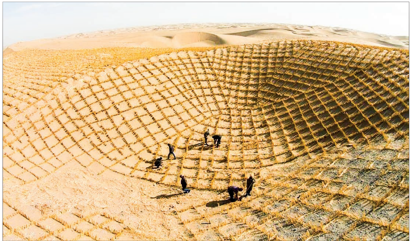
People fix straw checkerboards on sandy land in Qiemo County, northwest China’s Xinjiang Uygur Autonomous Region, 6 October 2014.
