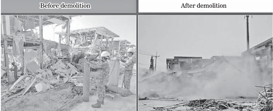
Demolition of illegally constructed two-storey residential buildings using explosives in KK Park area, Section (3).
