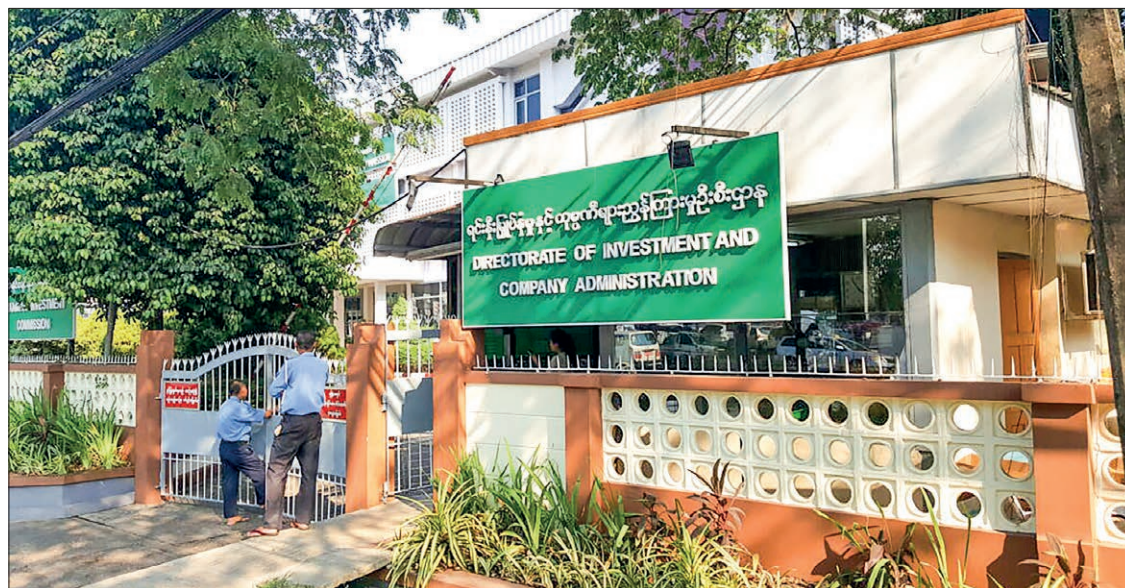
Front view of the DICA office in Yangon.
