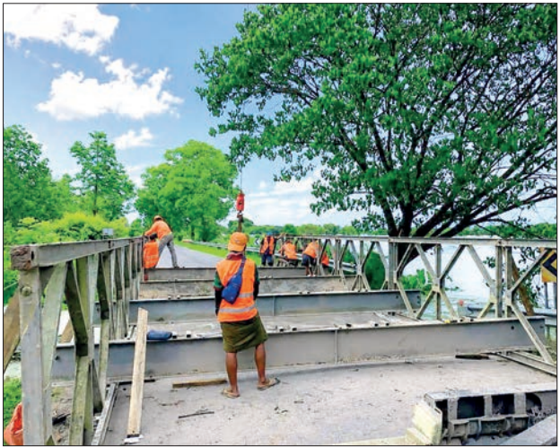
The Bailey bridge under construction for temporary use.
