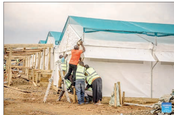
Workers build an Ebola treatment centre in Beni territory of North Kivu Province, the Democratic Republic of the Congo (DRC), on 22 July 2026. PHOTO: XINHUA
