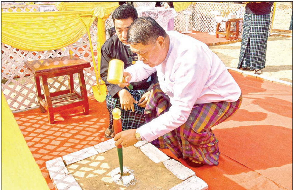
Chief Justice of the Union U Tha Htay drives the ceremonial pile to lay the foundation stone for the new Kachin State High Court building.
