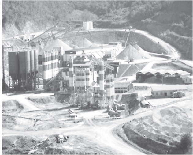
RCC Mixing Plant (Yeywa Hydropower Project)
