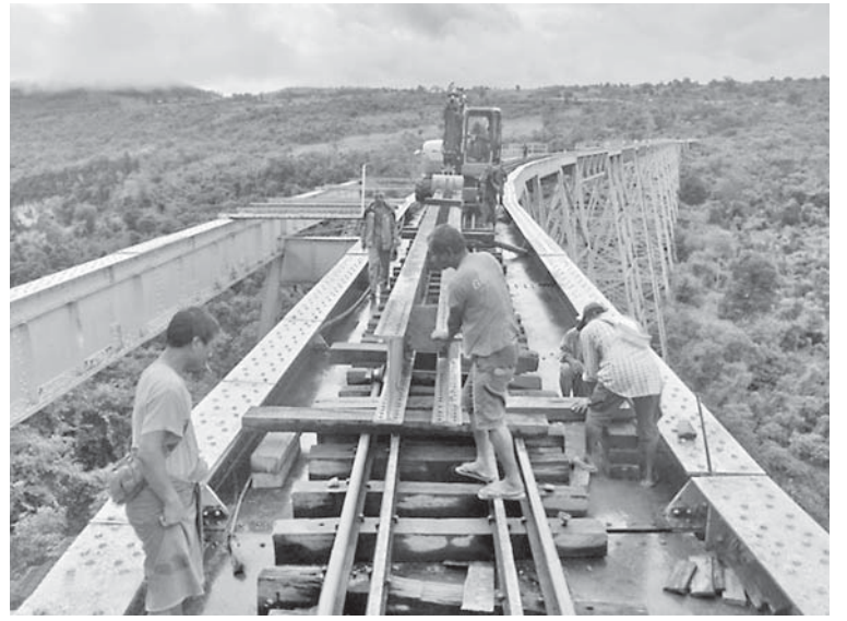
Workers repairing the damaged part of Goteik railway bridge.
