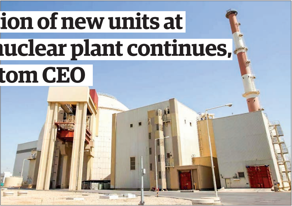
The image shows the Bushehr Nuclear Power Plant in Iran. PHOTO: SPUTNIK
