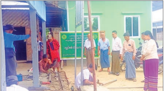
This photo shows youth trainees at practical welding work.
