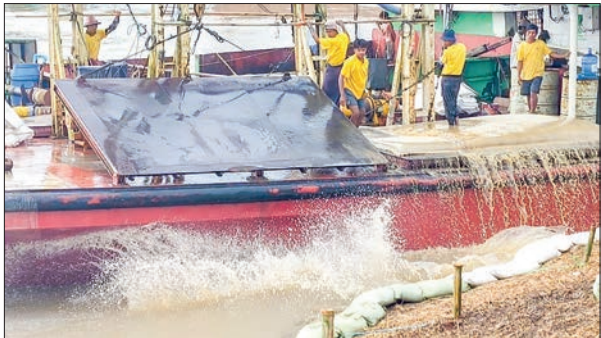
This photo shows temporary repair and reinforcement operations underway along the Ngawun River embankment.
