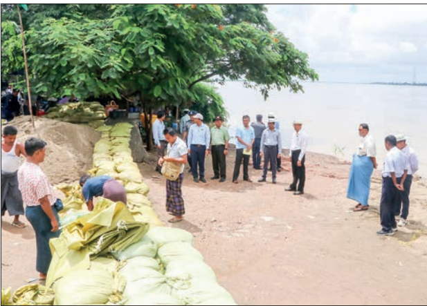
Photo shows volunteers stacking sandbags for flood prevention in Sagaing yesterday.
