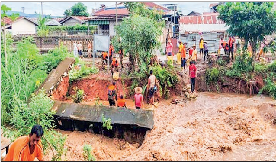
Photo shows a flood-affected area along Nampaw Creek in Nyaungpinkwin Village in Hsipaw Township, Shan State (North).
