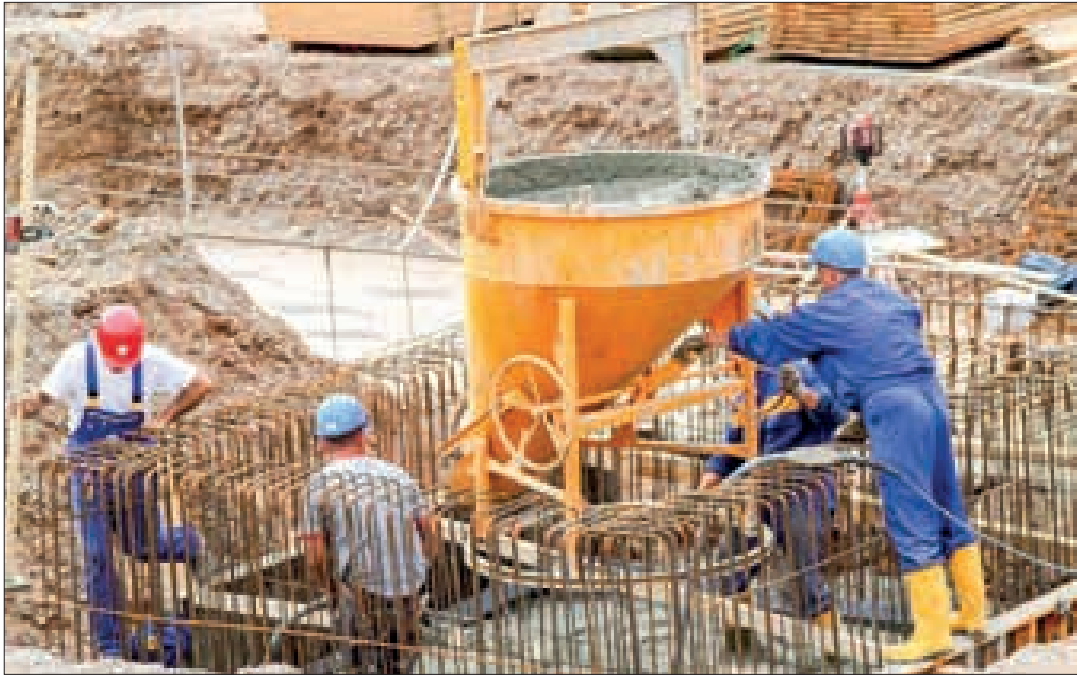
This photo showcases a construction site and its workers.
