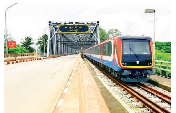
A DEMU train is pictured crossing the Thanlwin Bridge (Mawlamyine) over the Thanlwin River, Mon State, on the Yangon-Mawlamyine railway.
