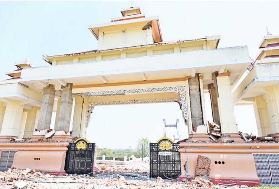
Damage at a Hluttaw gate.
