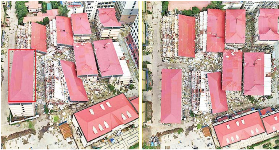
An illegal seven-storey residential building in the Shwe Kokko Area, Myawady District, Kayin State, where online scam gambling operations were conducted.
