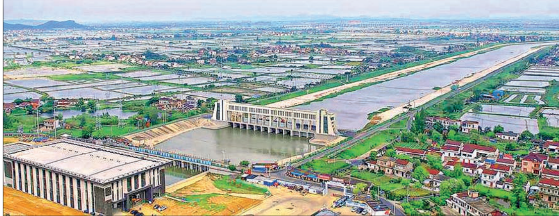
An aerial drone photo taken on 27 July 2025 shows the Fenghuangjing Pumping Station, which is part of the Yangtze-to-Huaihe Water Diversion Project, in Wuhu, east China's Anhui Province. PHOTO: XINHUA
