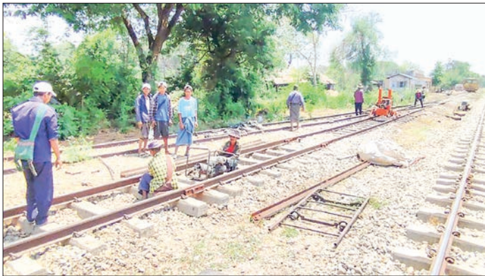
MR staff work on repairing damaged sections of the railway.
