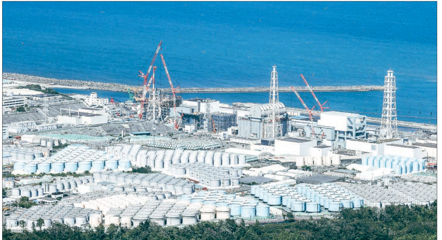
This aerial picture shows storage tanks used for storing treated water at TEPCO's crippled Fukushima Daiichi Nuclear Power Plant in Okuma, Fukushima prefecture on 24 August 2023. PHOTO: AFP
