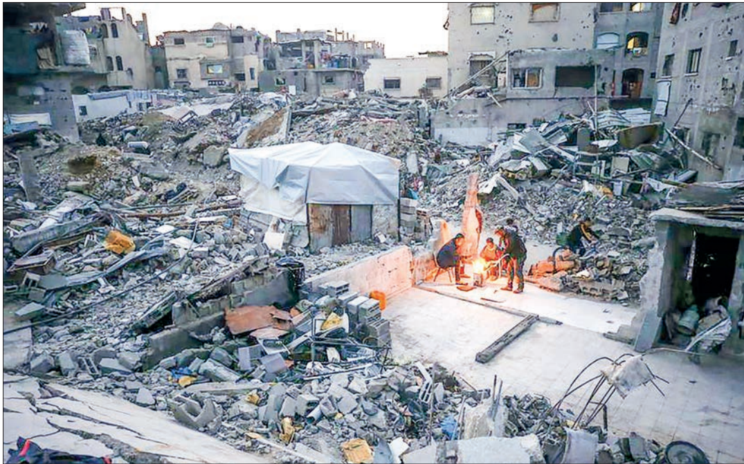
Palestinians are seen living among the rubble of destroyed houses in Jabalia in the northern Gaza Strip, 16 February 2025. (PHOTO BY MAHMOUD ZAKI/XINHUA)
