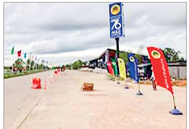
Photo depicts 76 th -Mile and 115 th -Mile Mini Rest Camps on the Yangon-Mandalay Expressway.
