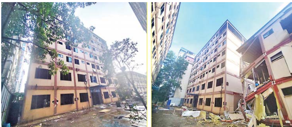
An illegal seven-storey residential building where online scam gambling operations were conducted in the Shwe Kokko area of Myawady District, Kayin State.
