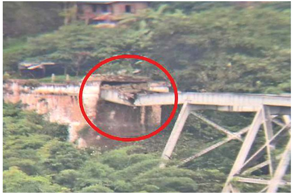
Photo record of TNLA terrorists planting and detonating mines to destroy the Gokteik Bridge.
