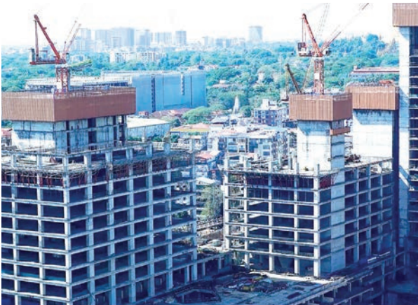
This image features a section of the stalled Yoma Central construction site in downtown Yangon.
