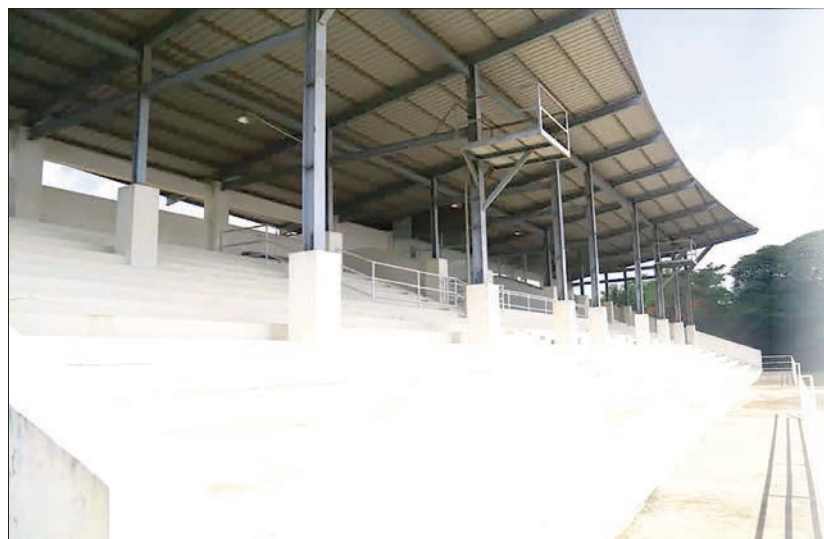
This photo depicts preparations underway at Grand Royal Stadium, which is set to serve as Hanthawady United's home ground. PHOTO: MNL
