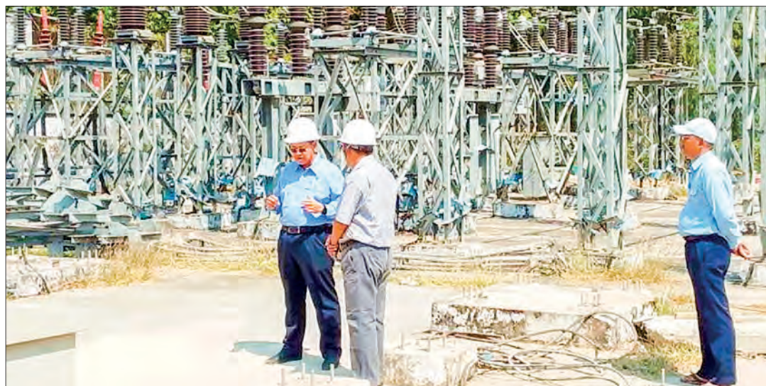
Officials inspect the power substation in Yangon Region.
