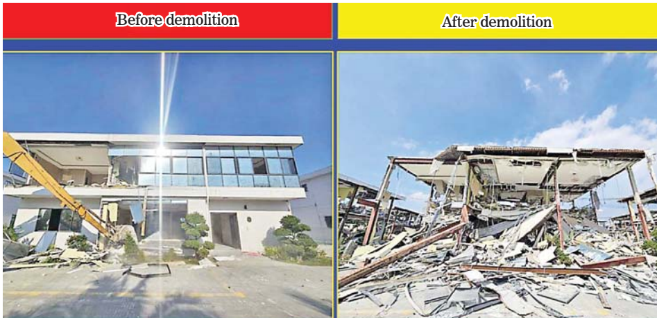
An illegally constructed two-storey residential building in Section 3 of KK Park area.
