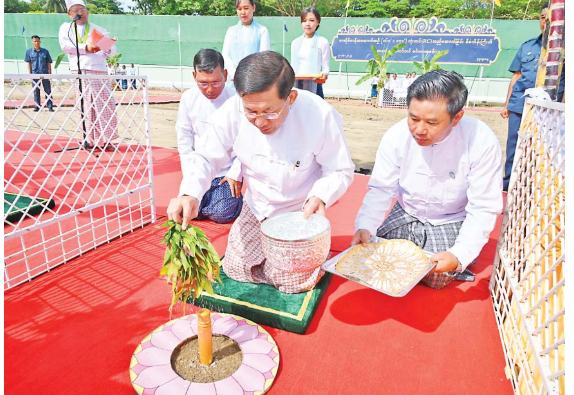
Senior General Min Aung Hlaing sprinkles scented water on a driven stake for construction of Sarso Beikman building.
