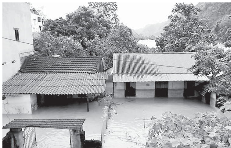
This photo taken on September 8, 2024 shows flooded buildings in Vietnam's northern province of Lang Son.
