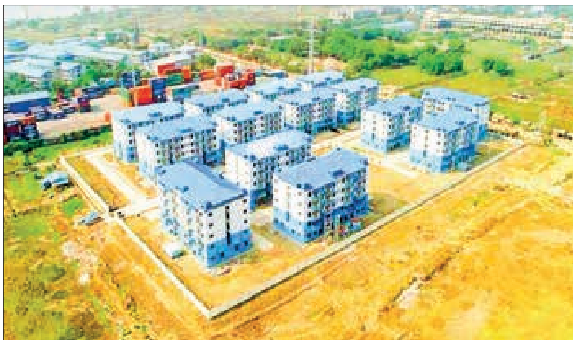
One of the Public Rental Housing projects in Yangon Region.
