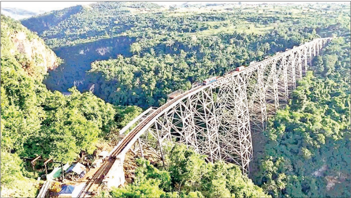
This photo shows the general view of Gokteik Viaduct.
