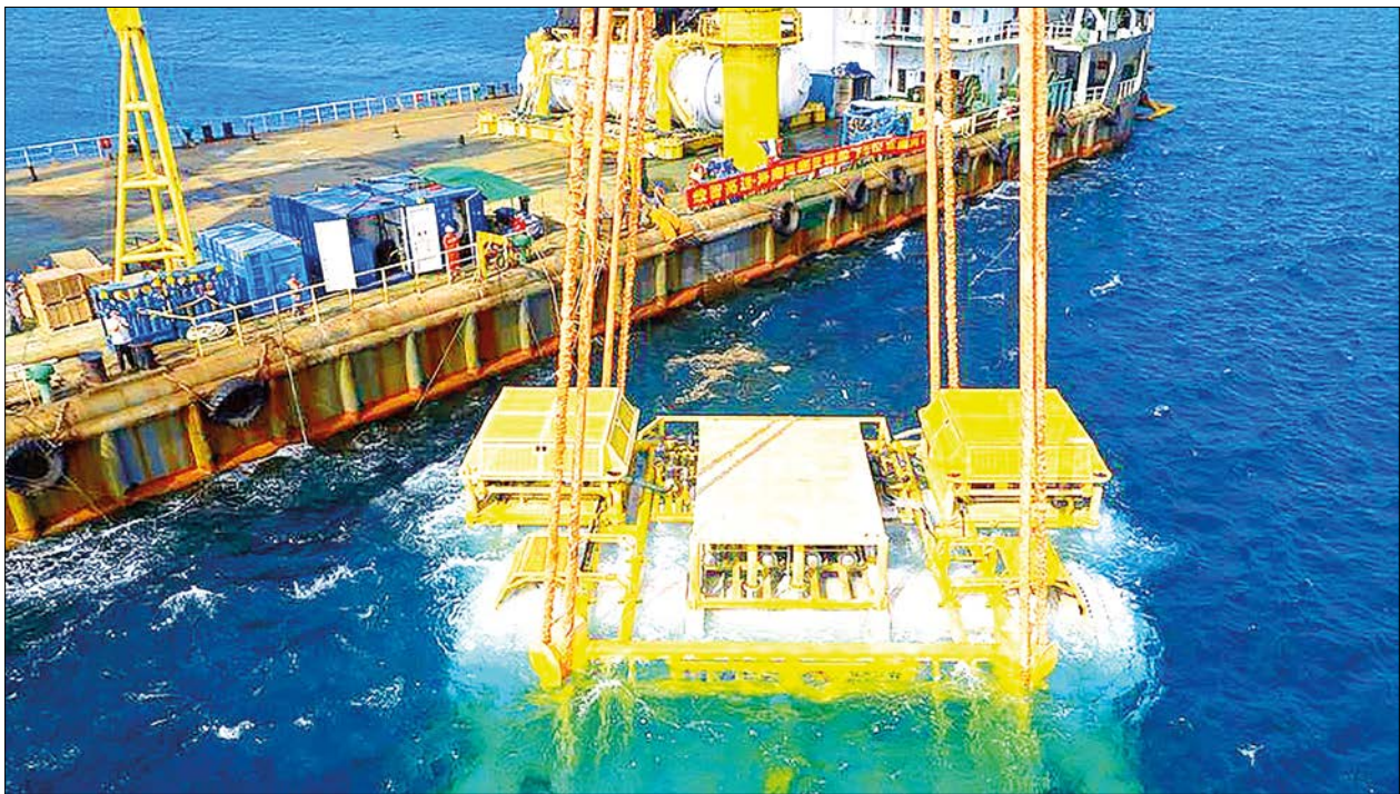
A drone photo taken on 18 February 2025 shows Hainan's commercial underwater intelligent computing cluster being lowered into the sea near Lingshui Li autonomous county in South China's Hainan province. PHOTO: XINHUA
