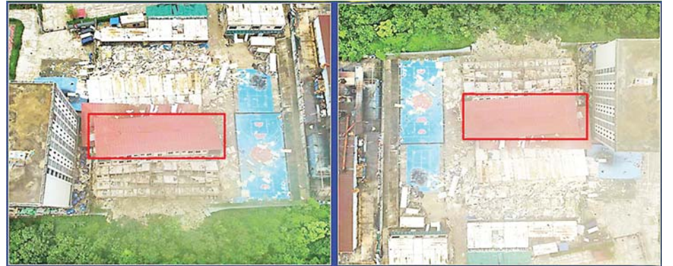
After demolishing an illegal nine-storey building used for online scam and gambling activities in the Shwe Kokko Area of Myawady District, Kayin State.
