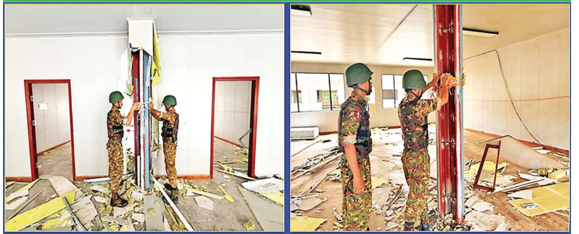
Preparing to demolish an illegal nine-storey building used for online scam and gambling activities in the Shwe Kokko Area of Myawady District, Kayin State with explosives.
