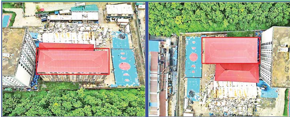
Before demolishing an illegal nine-storey building used for online scam and gambling activities in the Shwe Kokko Area of Myawady District, Kayin State.
