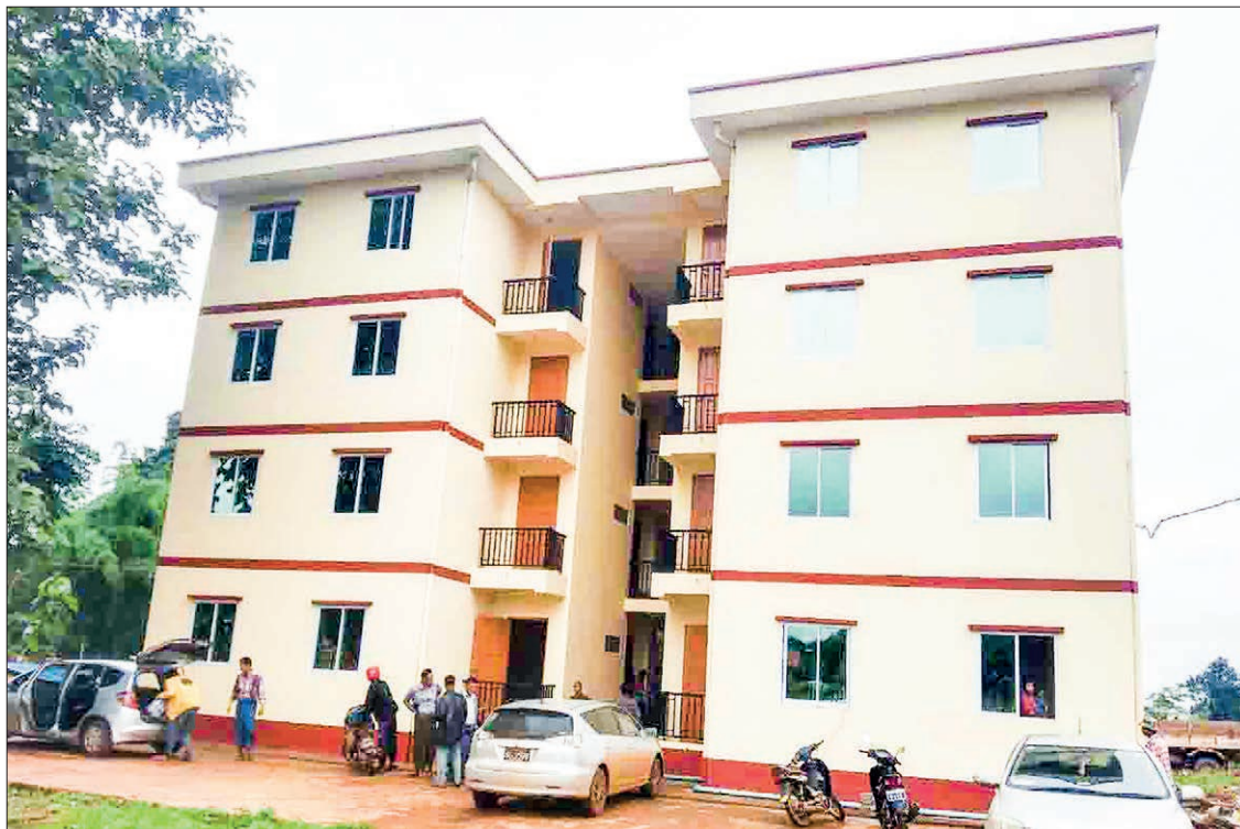
Already-renovated staff housings aim to accommodate staff in Hsihseng.
