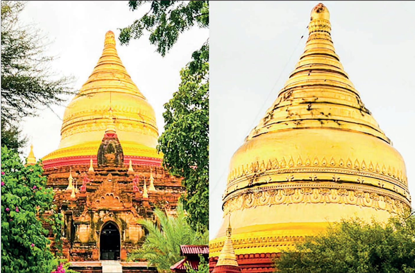
The photo shows Dhammarazika Pagoda struck by lightning in September 2023. PHOTO: DANM
