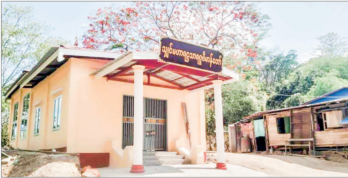
Mausoleum of scholar Shin Maha Ratthasara under construction.
