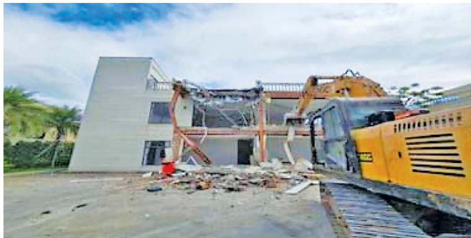
Documentary photographs showing the demolition of buildings in KK Park in Myawady.
