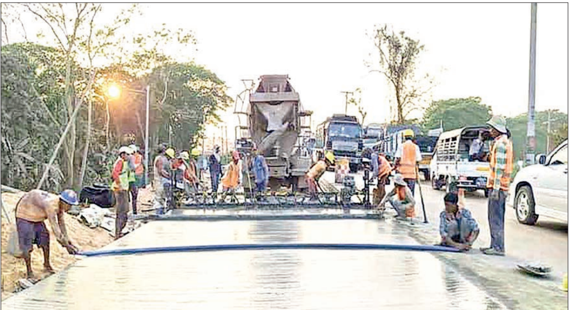
A view of some road sections where repair and maintenance work is underway on the Yangon-Pathein Highway.
