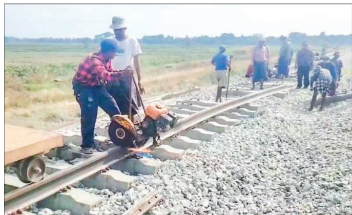
Workers repairing damaged rail tracks.
