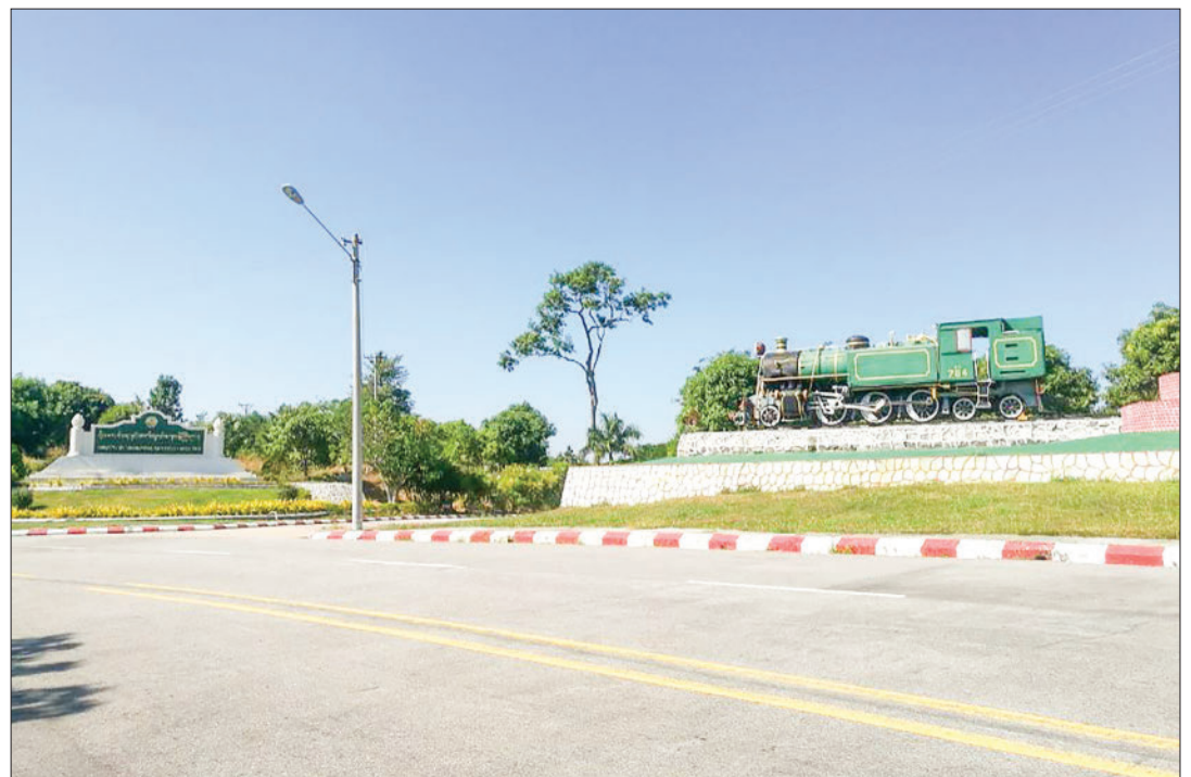
The photo shows Ministry of Transport and Communications office building in Nay Pyi Taw.
