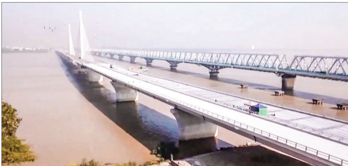
The photo shows the construction status of the Thanlyin Bridge No 3.
