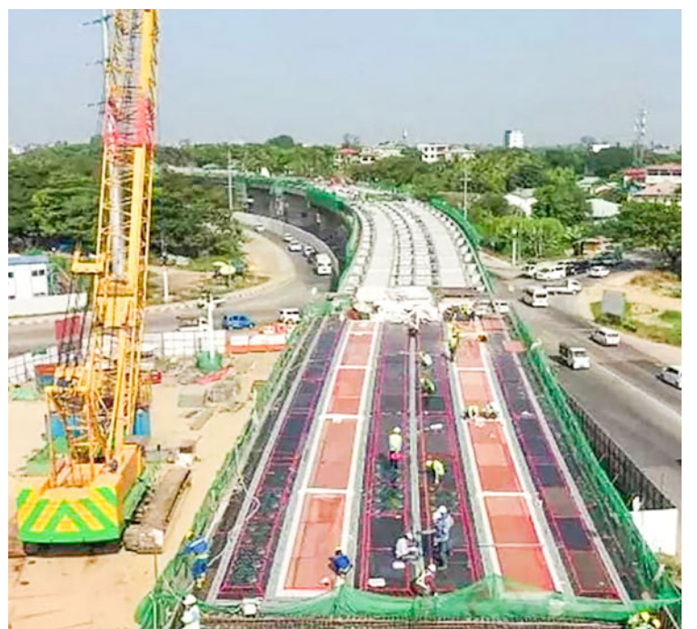
An aerial view of the construction progress of the Thanlyin Bridge 3.
