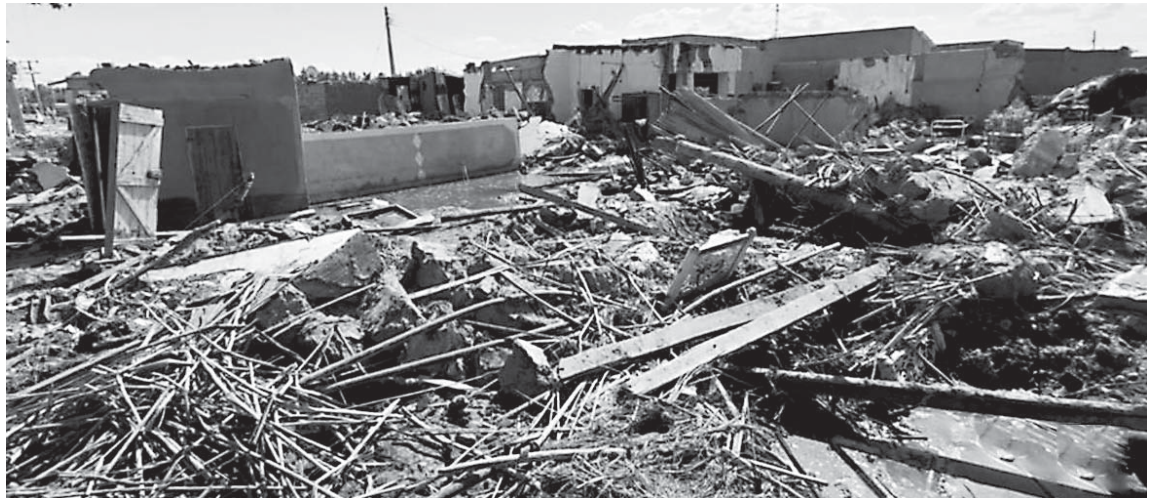
The photo taken on August 10, 2024 shows a flood-destroyed house in Abu Hamad city in the River Nile State in northern Sudan.
