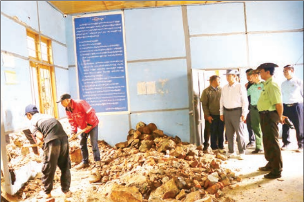
Deputy Minister Maj-Gen Kyaw Swa Oo and officials inspect repair and renovation work in Chin State.
