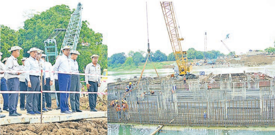
This photo shows the new Dokhtawady Bridge under construction.
