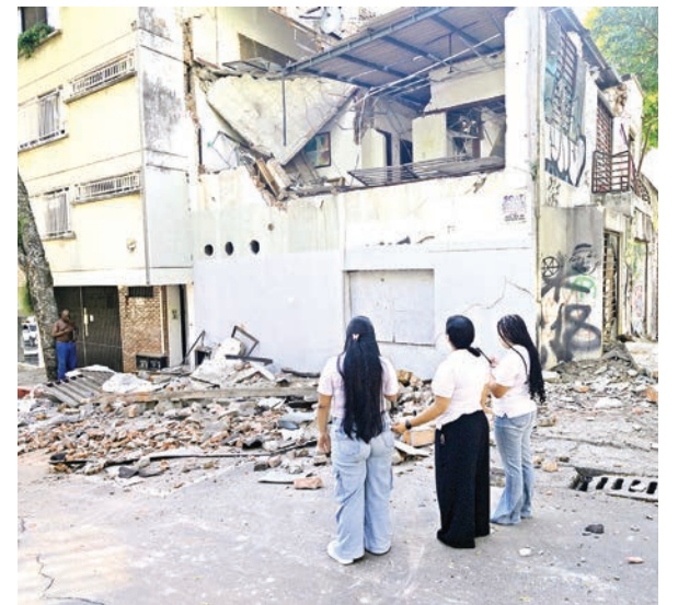
Women look at a damaged building after an earthquake in Cali, Colombia, on 10 August 2026. PHOTO: AFP
