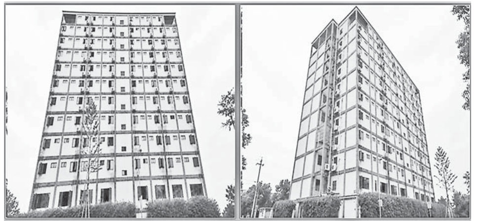
The 12-storey illegal building used in online scams/gambling to be detonated in Shwe Kokko Area in Myawady District in Kayin State. (Before demolition.)
