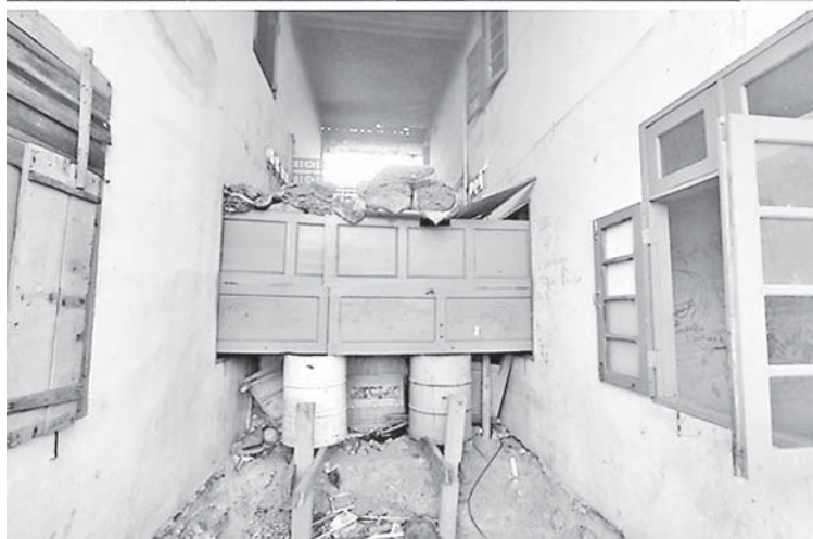
Bunkers constructed by terrorist insurgents at staff quarters in a police station in Thanlang.
