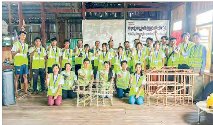
The On-the-Job Training (OJT) for carpenters in the restoration of traditional Inlay stilt houses.
