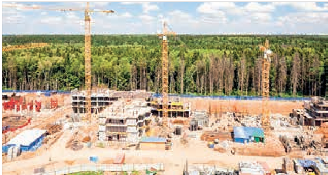
One construction site of the Russian Etalon Group. PHOTO: ETALON GROUP
