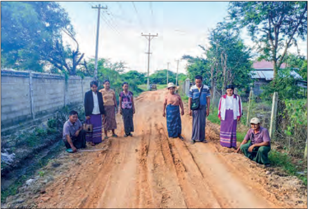
Officials oversee the implementation status of the road construction project in Yamethin Township.
