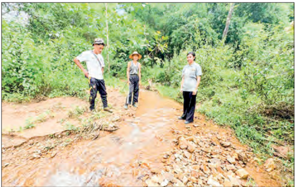
Officials inspect an ongoing spring water supply project in Kehsi Township in southern Shan State.
