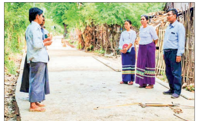
Officials of Department of Rural Development inspect progress of concrete road in Kyaukpadaung Township on 7 June.
