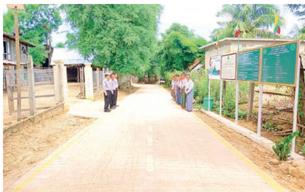
Officials and locals are seen alongside the completed concrete road in Magway Township.
