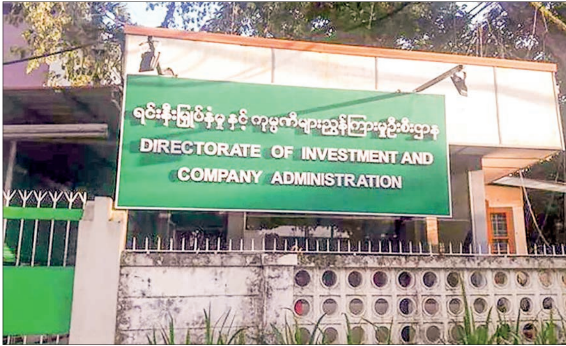
The office of the Directorate of Investment Company Administration (DICA) in Yangon.
