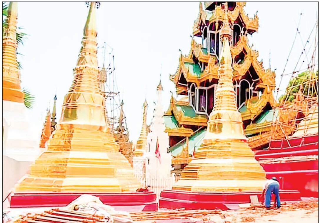
The photo shows maintenance works at Shwedagon Pagoda.
